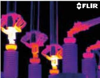
*Thermal inspection of a high voltage installation.*
