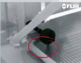
A leaking pressure gauge.
